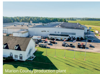
Marion County production plant
